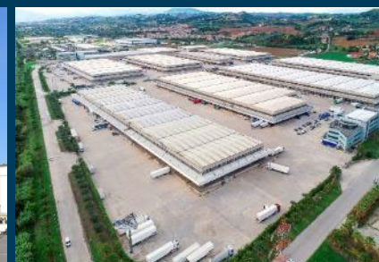
Centro Logistico Orlando Marconi (CLOM) Monteprandone, Italy
