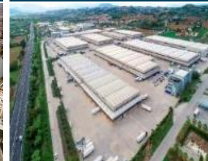
Centro Logistico Orlando Marconi (CLOM) Monteprandone, Italy
