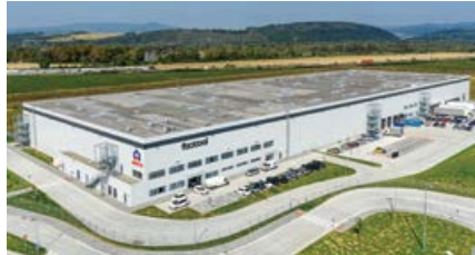
2 Nove Mesto ONE Industrial Park I, Beckov
