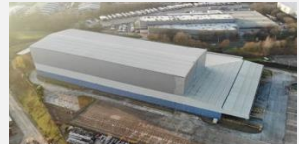
The Cube, United Kingdom Light industrial / logistics
