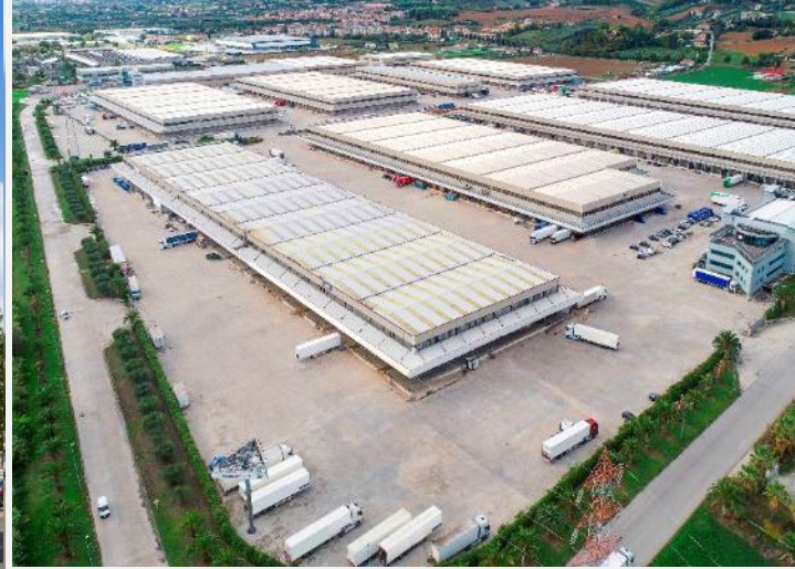
Centro Logistico Orlando Marconi (Montepandone, Italy)
