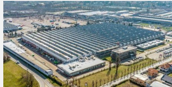
Via dell'Industria 18, Italy Light industrial / logistics
