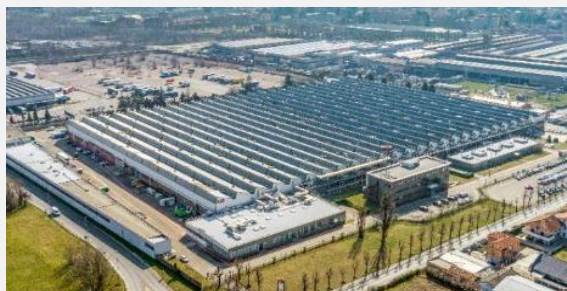
Via dell'Industria 18, Italy Light industrial / logistics
