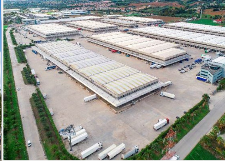
Centro Logistico Orlando Marconi (Montepandone, Italy)
