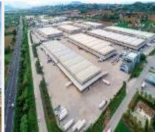
Centro Logistico Orlando Marconi Montepandone, Italy
