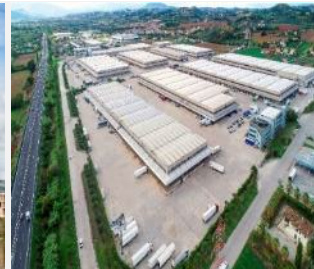
Centro Logistico Orlando Marconi Montepandone, Italy
