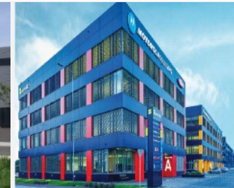
Green Office Kraków, Poland
