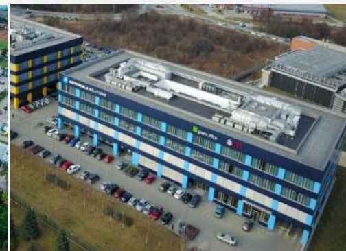
Green Office (Kraków, Poland)
