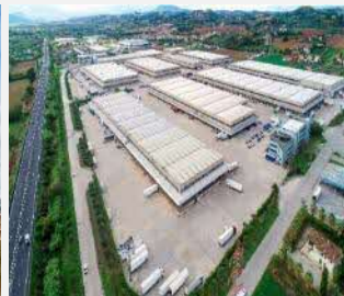
Centro Logistico Orlando Marconi Montepandone, Italy
