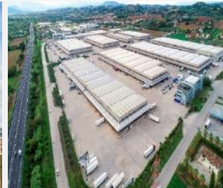
Centro Logistico Orlando Marconi Montepandone, Italy
