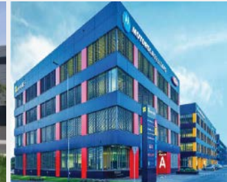
Green Office Kraków, Poland
