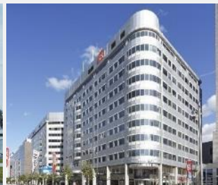
Central Plaza Rotterdam, The Netherlands
