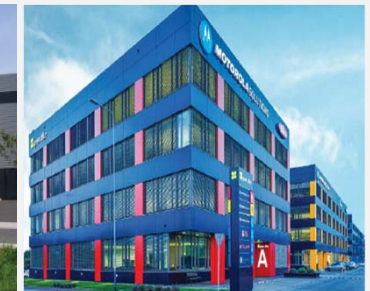
Green Office Kraków, Poland
