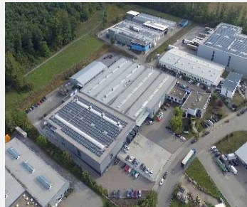
Bretten Pforzheim, Germany
