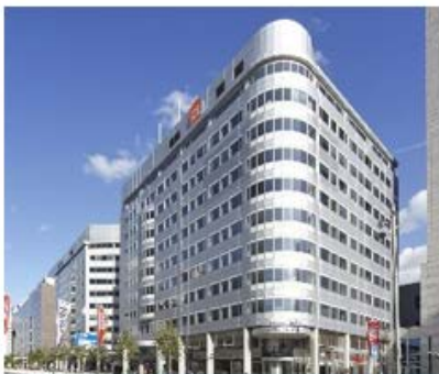
Central Plaza Rotterdam, The Netherlands
