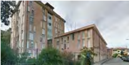
16. Padova, Via Brigata Padova 19, Padova
